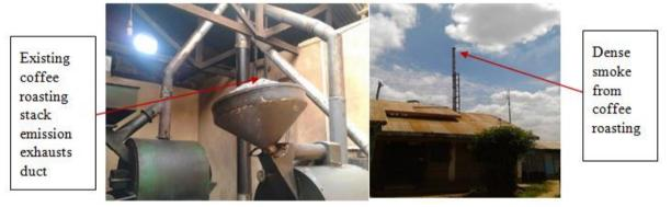
Fig.1. Roaster exhaust ducts joined to one main exhaust duct extending outside the roof
