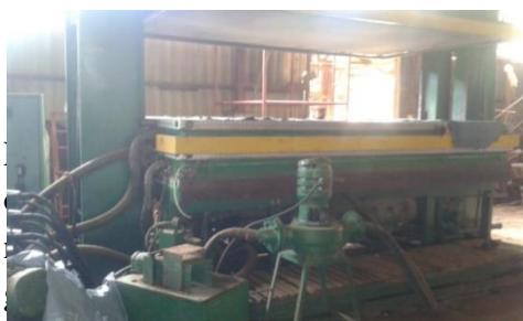
Figure 0.7: The broken-down vacuum drying machine. Source: STL
