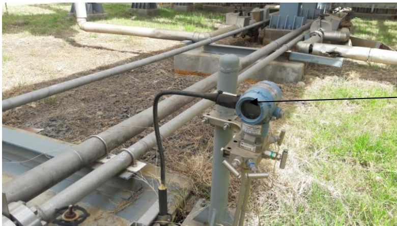
Figure 3. 3: Steam washing flow meter (4-6 tons/hr)
