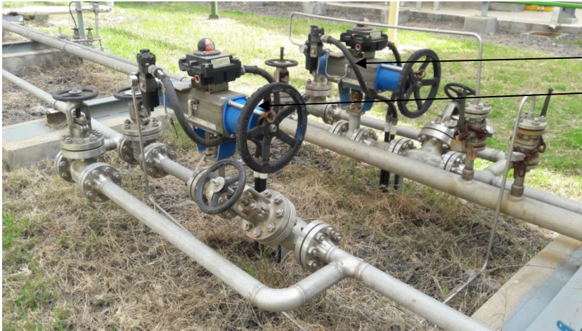
Figure 3. 1: Steam washing valve arrangements
