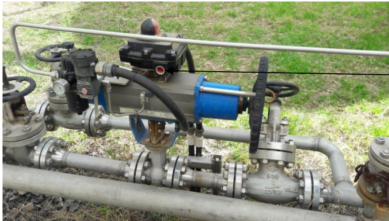
Figure 3. 2: Steam washing valve closed before the experiment
