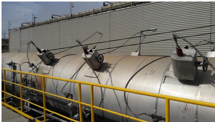
Figure 3. 4: Steam washing Spray nozzles
